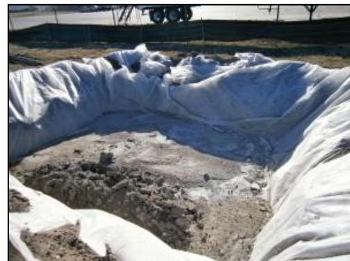
Plate 4-2 Concrete washout area
