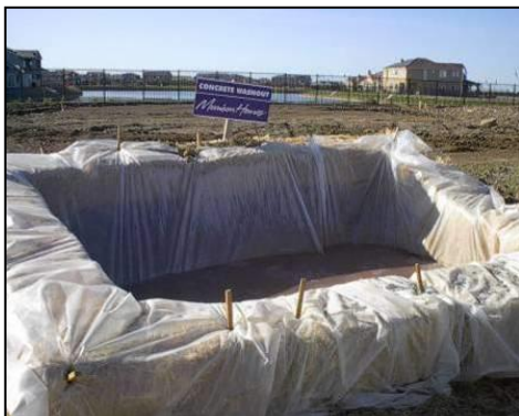
Plate 4-1 Concrete washout area
